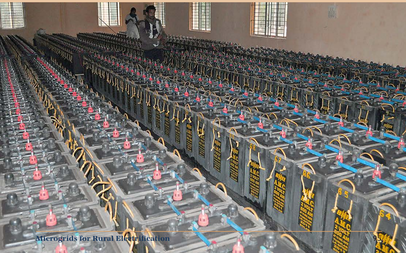
Onsite water distillation tables (above) to service its massive battery system (below) helped WBREDA maintain reliability on its solar PV microgrid in Sagar Island, West, Bengal, India
