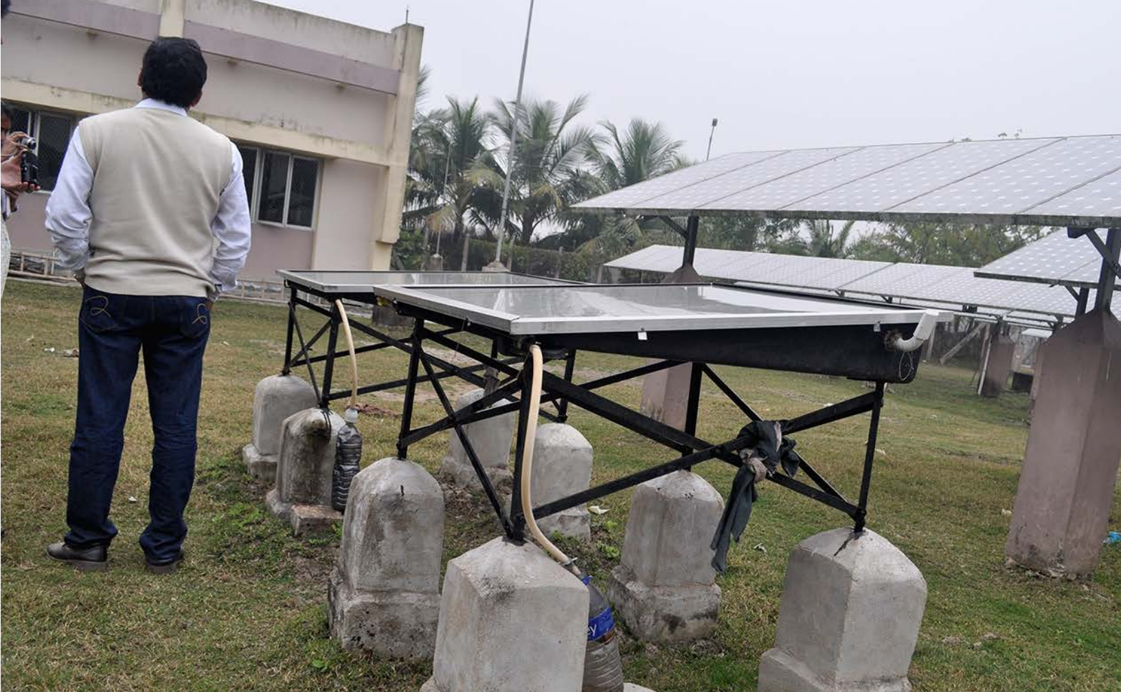
Onsite water distillation tables (above) to service its massive battery system (below) helped WBREDA maintain reliability on its solar PV microgrid in Sagar Island, West, Bengal, India
